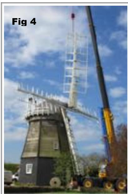
In May 2013 a large crane was hired to remove the damaged pair of sails (fig 4). This revealed the extent of the rot inside the stock (fig 5). But more seriously, in removing sails I and II it was discovered that sails III and IV were also badly rotten and would also need urgent replacement, triggering a major rethink of the planned restoration programme.
